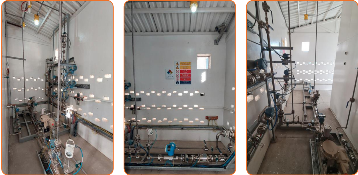
Figure 6 - Fabricated fuel mixing skid
